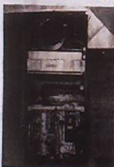
EXPOSED VIEW OF HEAT PUMP shows unit dug ground at right. Compressor is at bottom left, cooling tank at bottom right and flow air is top center. Unit is 4 feet 3 inches tall, occupies 6 1/2 square feet of floor space.
