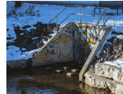
Storm and sewer
