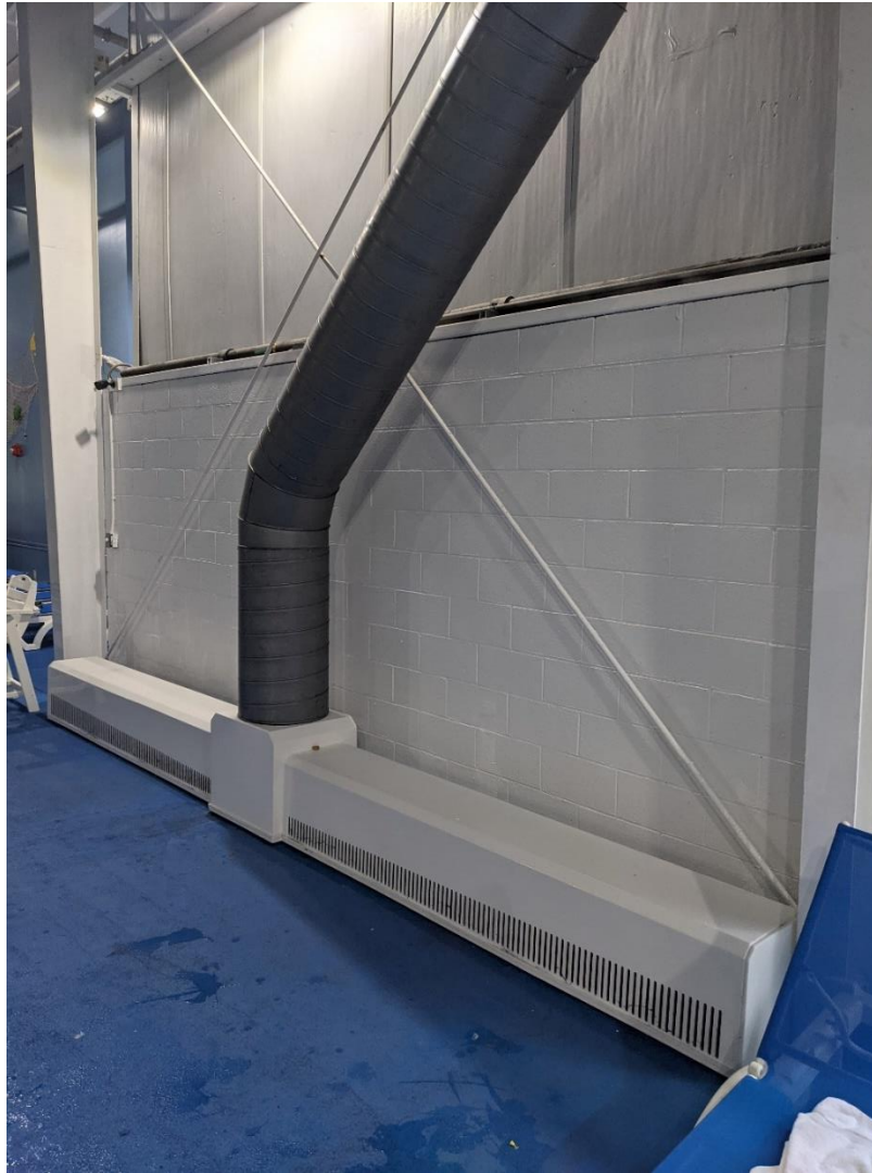
Retrofit of deck bench exhaust
