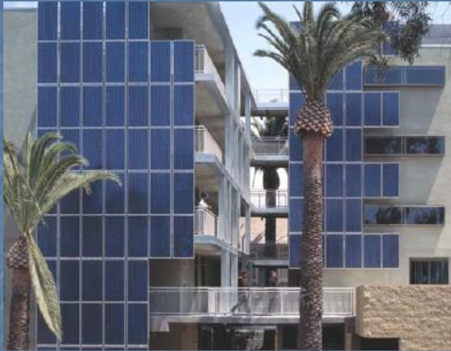
Clearview Court. 100% PV gas microturbine w/HR
